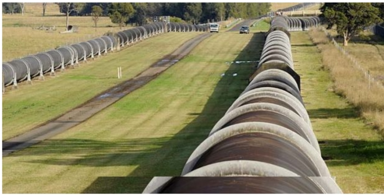
Maintenance ... a pipe from Warragamba Dam. Photo: Adam Hollingworth
